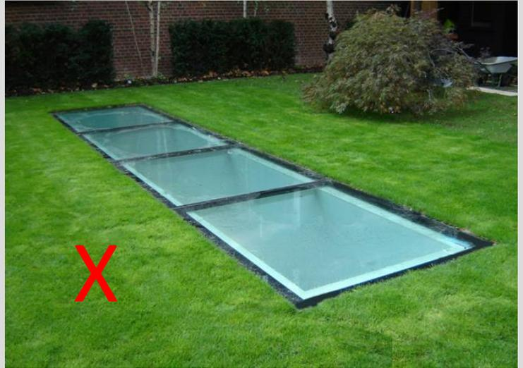
Figure 8 (above): Photo showing an inappropriate location for roof lights in a garden
