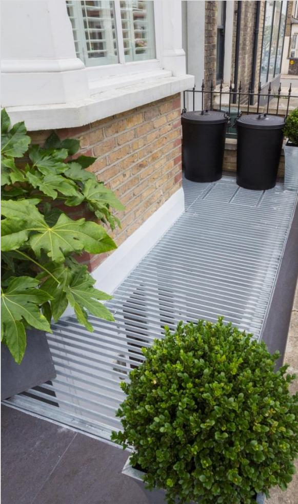
Figure 7 (left): Photo showing a flush lightwell that allows light to penetrate to the floor below
