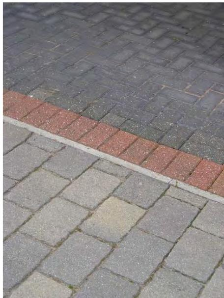
9.1.012 Value for money: The traffic calming scheme around Highbury Fields, includes dropped kerbs instead of raised table crossing, allowing for simple drainage, where the alternative would have required a 75m+ long new drainage channel to link to existing services. The preferred option was identified as a result of sub-surface investigations at an early stage.
